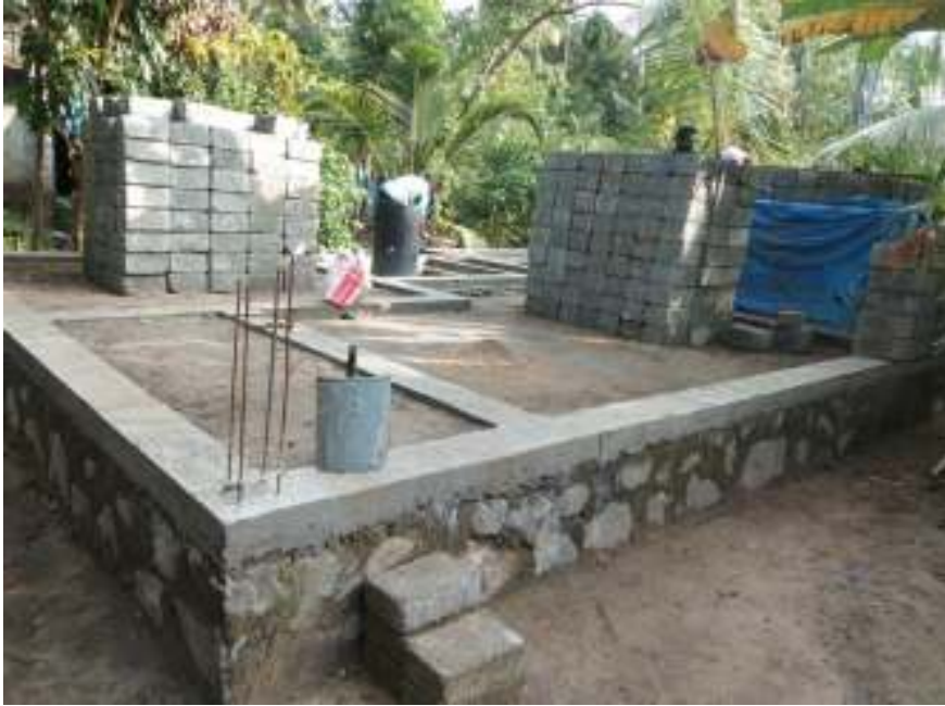
completed Basement before flood
