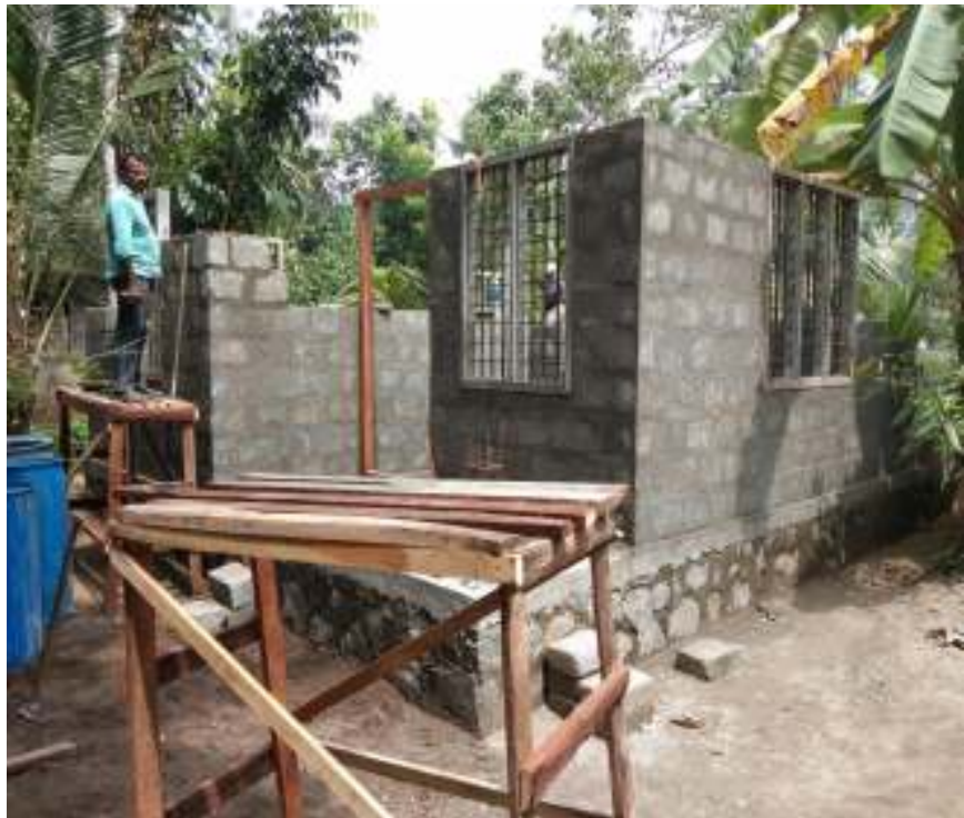
Completed the Work Till the Lintel level
