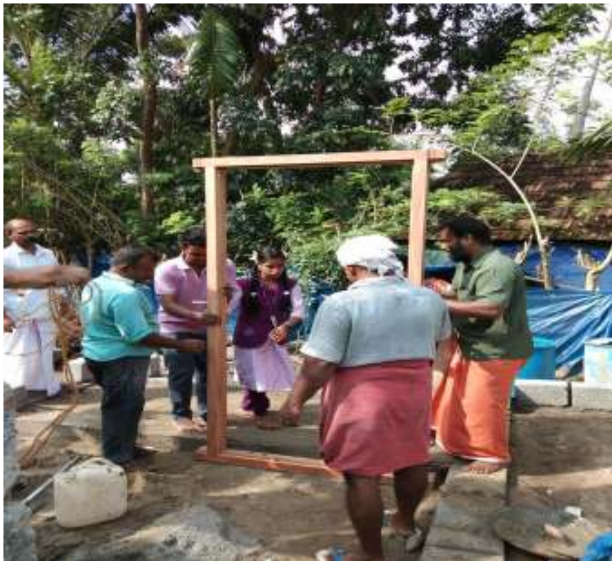
Work Begins After Flood-
