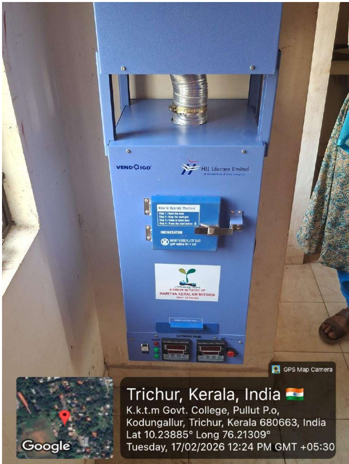
Installation of Incinerator in lady's Amnity centre .17.2.2026
